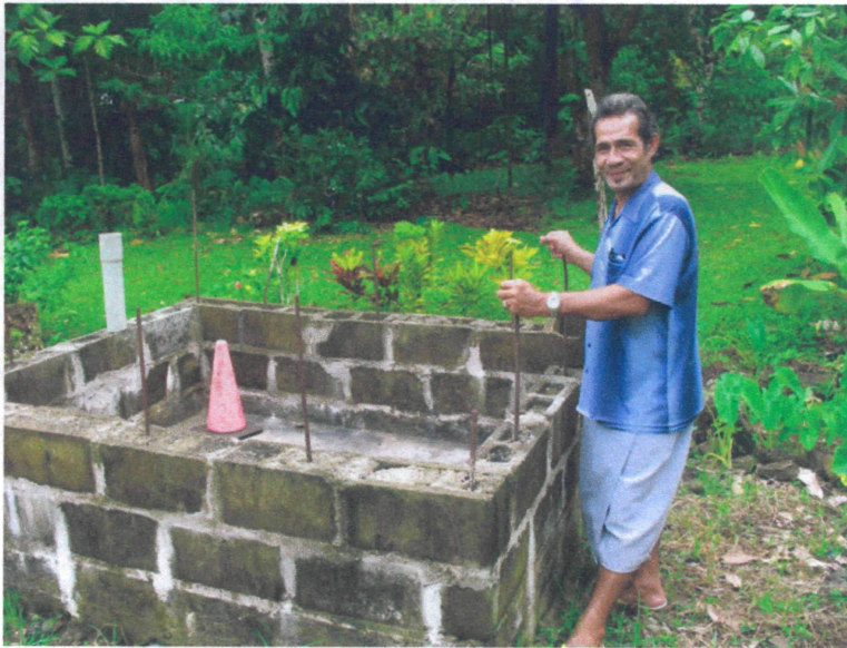
Figure 1. Here is my tank under construction. Its final dimensions will be 6'x6'x4'.
