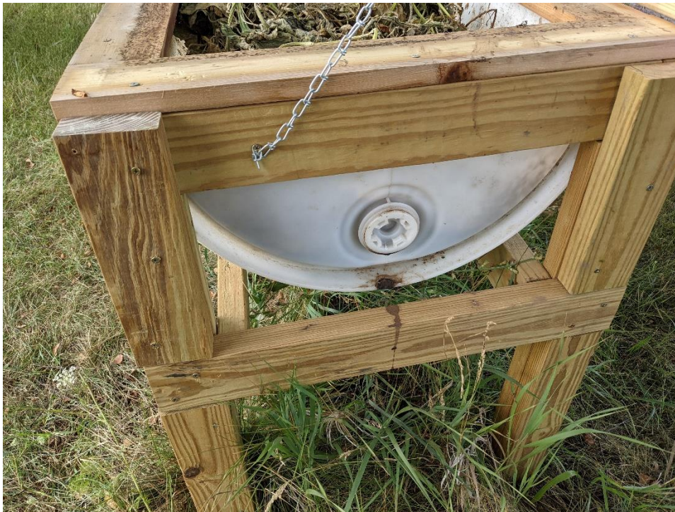
Last two 38-inch 2x4s connection to leg base (view from the top)
