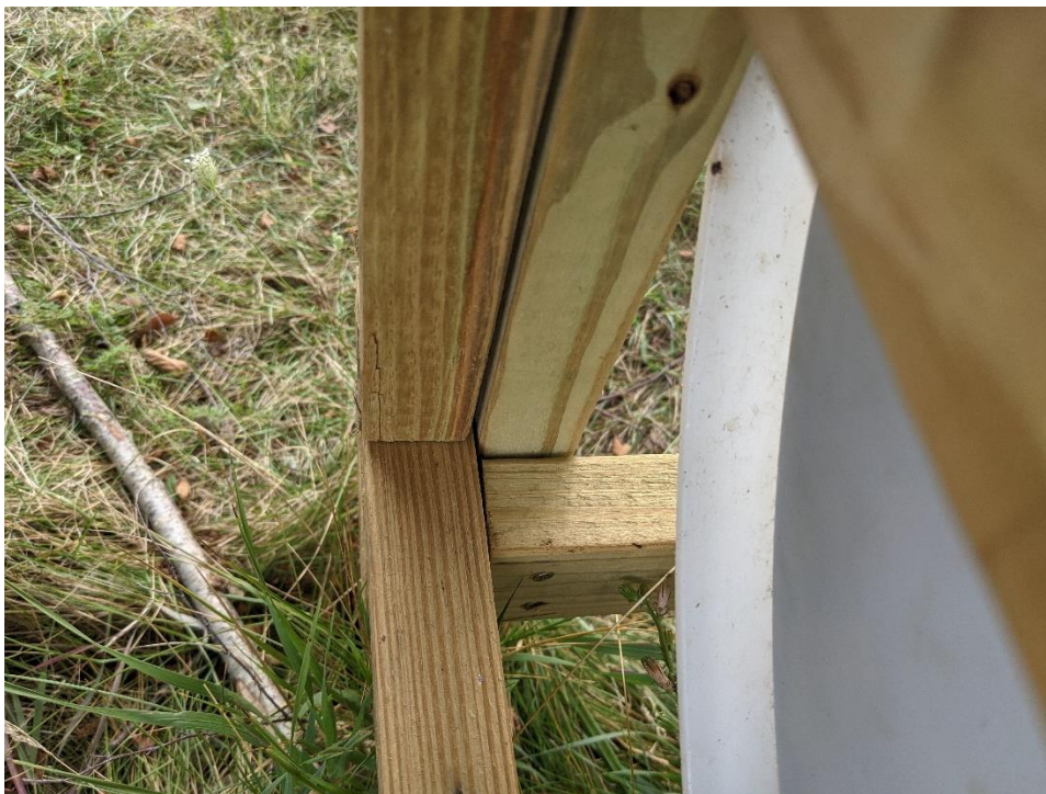
Top of ramp and frame connection within bin
