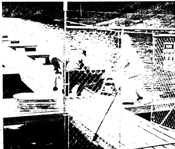
The "T" shape keeps a floating dock steadier.
