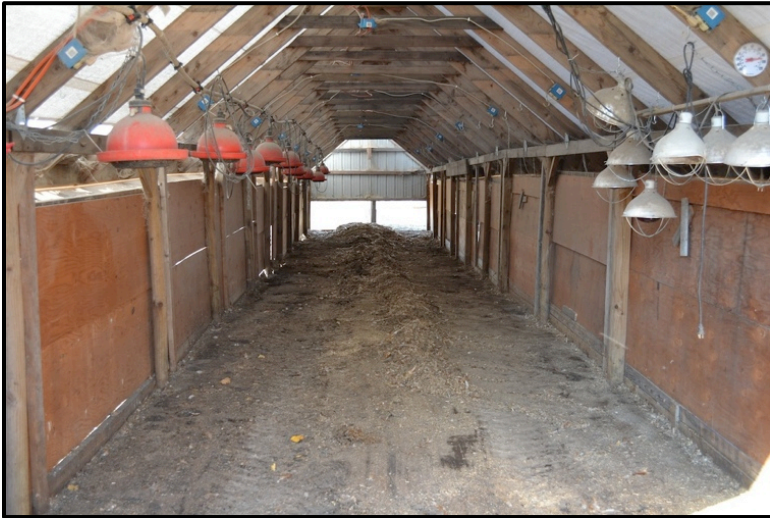
Water Fountains and Heat Lamps Hung High in Preparation for Cleaning Building
