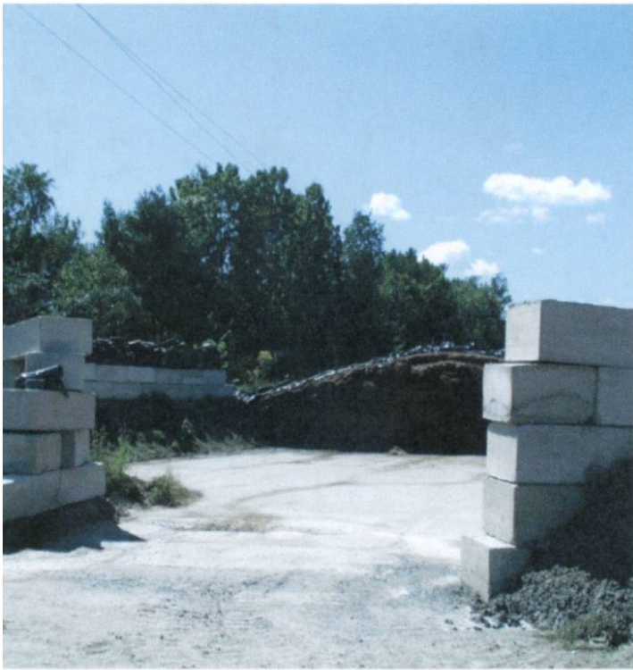
New Silage Storage Facility 09-09-03
