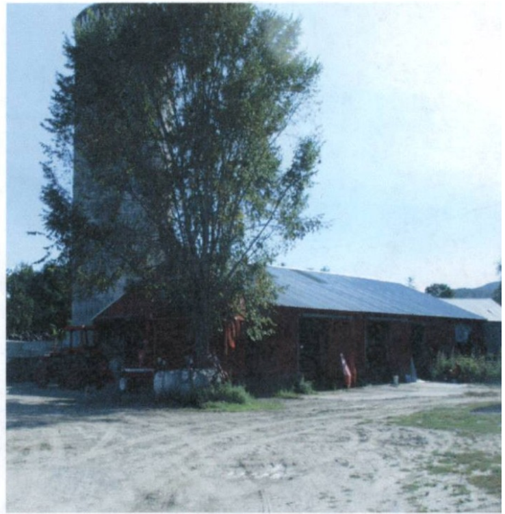
Farm Buildings & Silo 09-09-03
