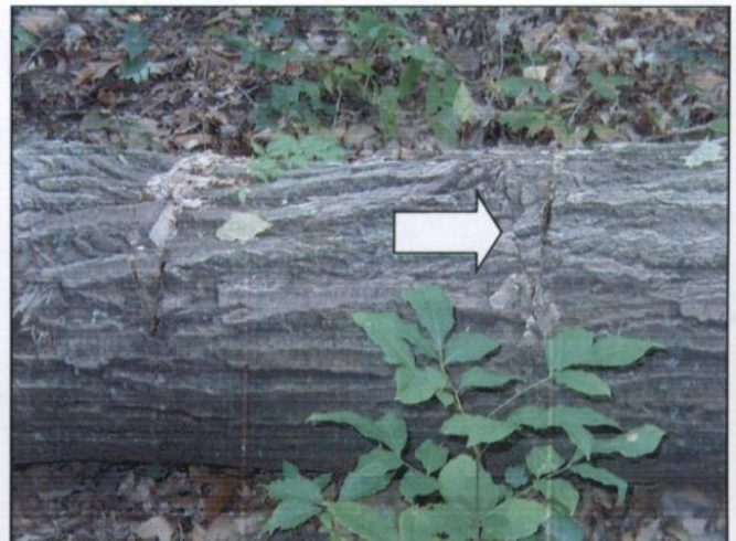
Photo 4—Arrow points to wedge cut by chainsaw. This method proved to be productive and less labor intensive.
