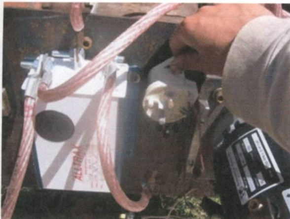
Installing the Contactor
