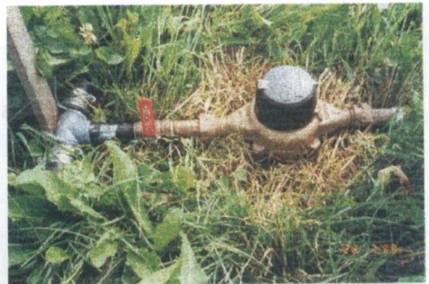
Figure 9. Watering connection point at the main distribution pipe serving the study paddocks. A 0.75 inch Neptune water meter has been inserted at this site for the project.
