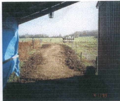
Figure 3. Improved section of main laneway leading from milking parlor.
