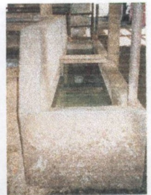
Figure 4. One of seven water troughs located in freestall barn.
