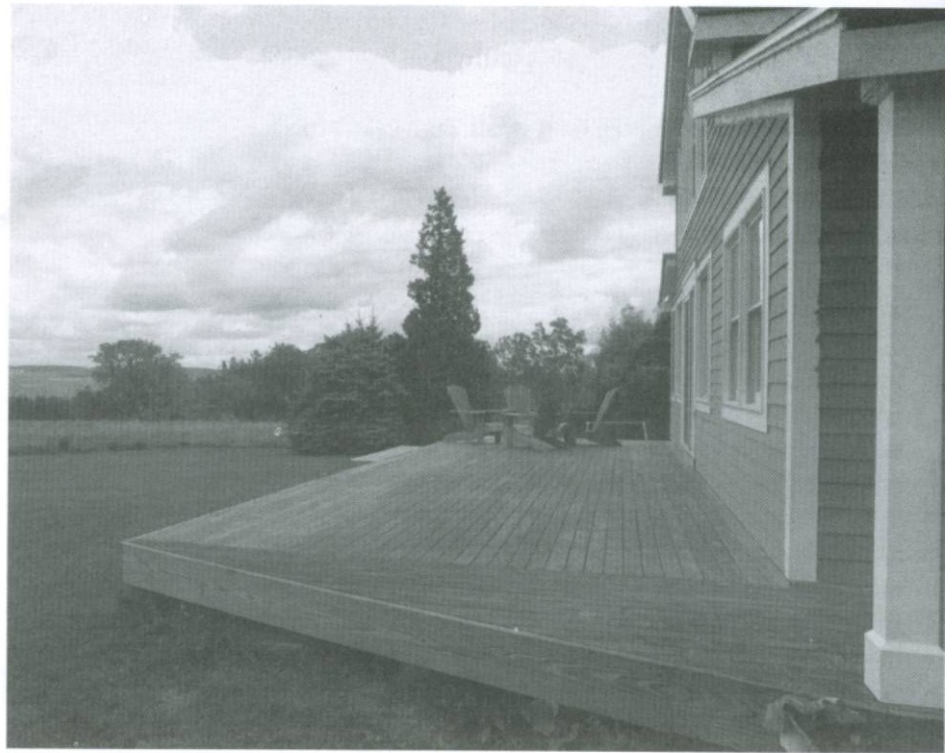
A locust deck in Trumansburg, NY. Photo by Mike Hopiak
