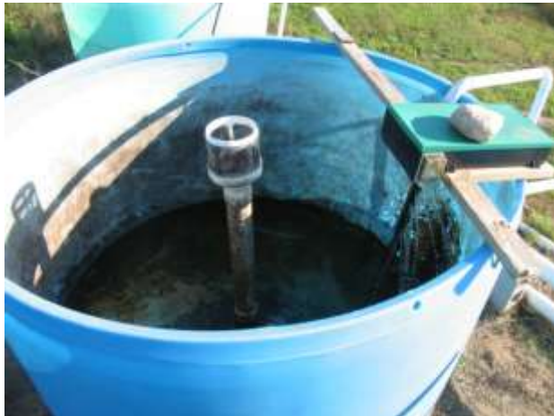
Typical overhead view showing incoming water, center overflow, and belt feeder. Bottom drain not shown collects waste
