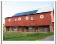
Solar panels, on the southfacing roof of their 1840s barn generate electricity for their entire farm (house and outbuildings). On most days, they even produce more electricity than the farm operation needs and the Bocks are able to sell the excess back to their supplier. was sponsored by the Rodale Institute and Penn State, receiving support from SARE as well as the Kellogg Foundation and the Towards Sustainability Foundation.
