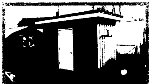
Photo 7 - Building for Backup and Greenhouse Manifolds
