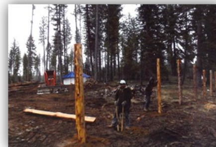
Building the fence around the berry field
