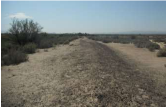
5.a) Large structures along the main channel (example Ryan dike in the photograph)
