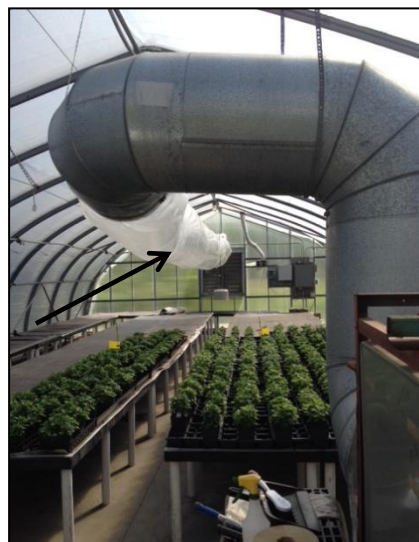
Fig. 19. An overhead heat system that would be more efficient if re-located under the benches. It should be noted that under-bench locations may require increased need for watering.
