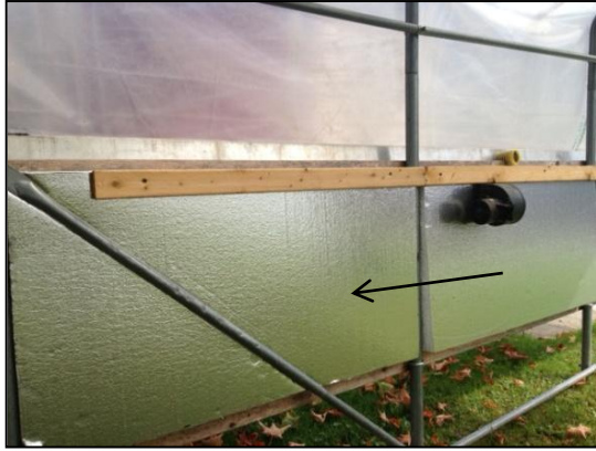
Fig. 5. Aluminum-faced foam board to insulate the end and side walls eliminates the need for the poly layer.
