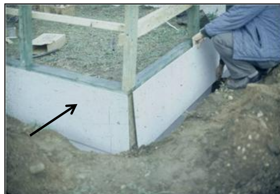
Fig. 8. Insulate the perimeter foundation with foam board.
