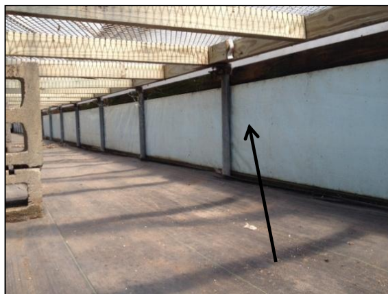
Fig. 9. Foam board insulation on a knee wall from the floor up to bench height covered with poly. Use of aluminum-faced board may eliminate need for the additional layer of poly.
