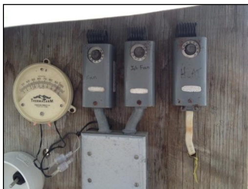
Fig. 18. Older thermostats that should be cleaned annually.
