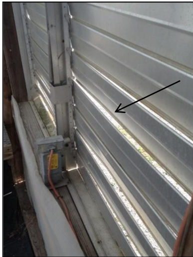
Fig. 7. Improperly adjusted louvers. Note the cracks (indicated with arrow) where heat can easily leak to the outside.
