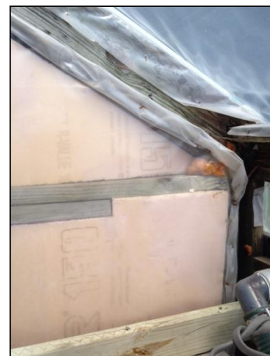
Fig. 10. Insulated and poly-covered end wall.
