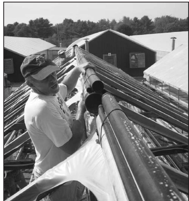
Figure 4. Installation of bubble system by consulting engineer and UVM personnel. Photos by Margaret Skinner
