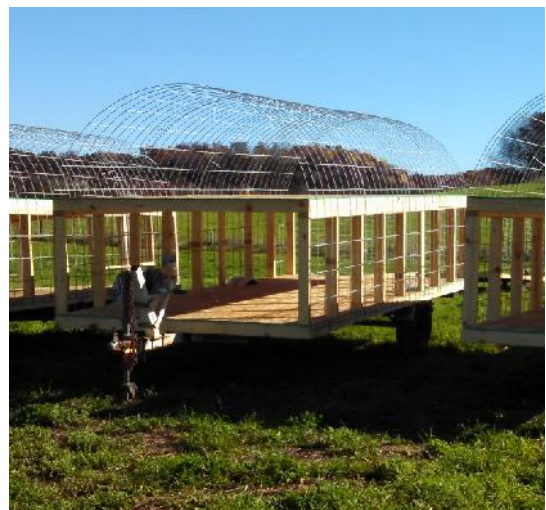
Double Deck shelter prior to covering
