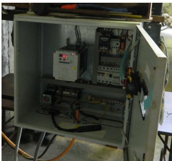
Figure 14. Side-mounted control panel.
