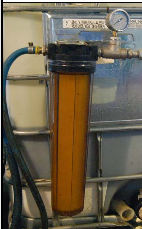
Figure 2.4.7: Cartridge filter with clear housing used as final filter for fueling with straight vegetable oil.
