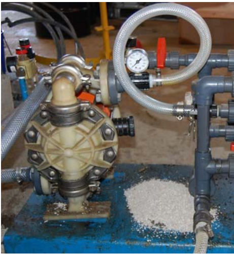
Fig. 10: Air operated diaphragm pump on filter press
