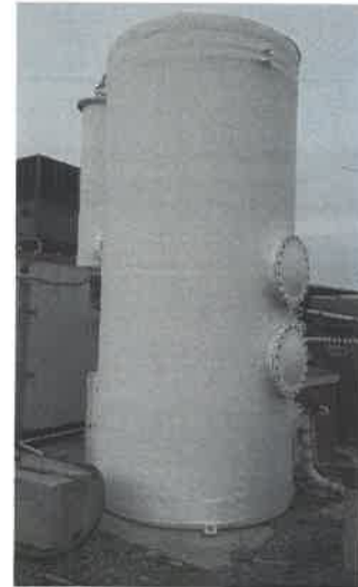
Figure 1. Spruce Haven Biological Trickling Filter
