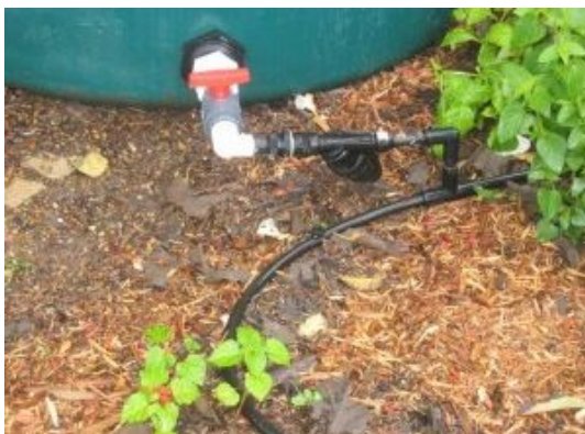
Spigot with valve on drip irrigation system.
