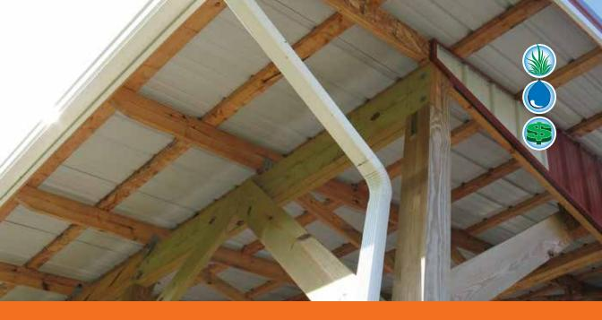
**Roof Runoff System** A system for collecting, controlling and disposing of runoff water from non-residential farm buildings.
