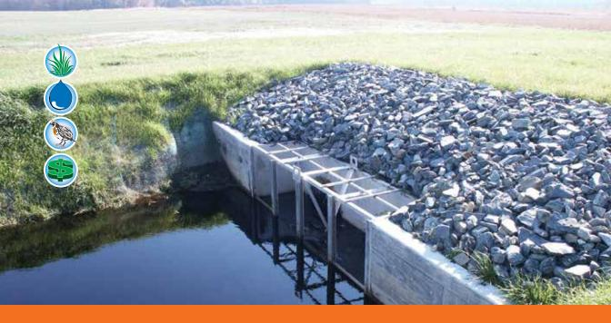
**Grade Control Structure** Earthen, wooden, concrete, or other structure built across a drainageway or gully to control and reduce water flow.
