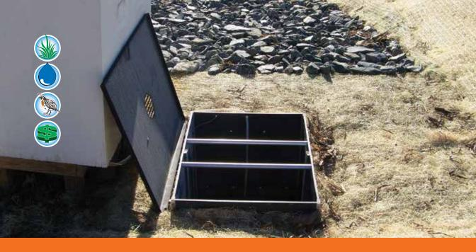
**Water Control Structure** A structure in a water management system or drainage channel that conveys water, controls the direction or rate of flow, maintains a desired water surface elevation, or measures water.
