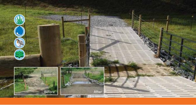
**Livestock Stream Crossing** A stream crossing provides a hard, stable area where cattle or equipment can cross a stream without damaging the streambed or banks.
