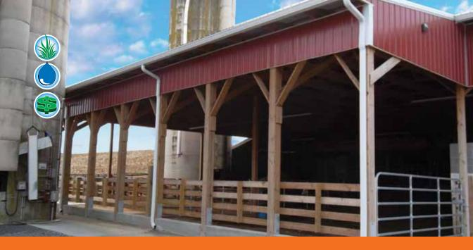
**Roofs and Covers** A roof structure placed over a heavy use area to divert clean water from animal management areas such as barnyards or feedlots.
