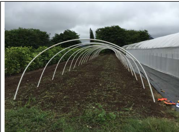
Hoop structure with rebar and PVC pipes.
