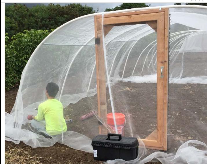
Install a door and adjust the height of PVC structure, then secure the PVC to rebar using self-tapping screws. Cover the structure with insect netting.
