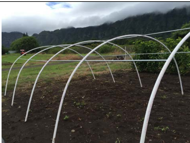
EMT conduits provide structural support between PVC pipes.
