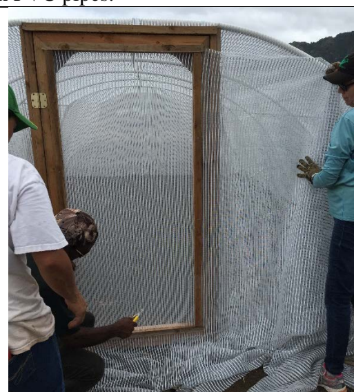
Staple netting to the door before cutting off excess netting.
