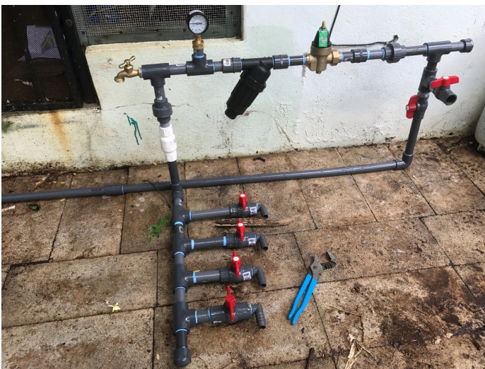
Figure 5 Components of a Multi-zone Drip Systems control manifold note pressure regulator, filter pressure gauge, backflow preventer and shut off valves/hose link for individual zones, among others.
