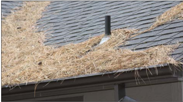
Photo: John O’Conner, © Oregon Department of Forestry Clean the roof to keep embers from igniting tree litter.
