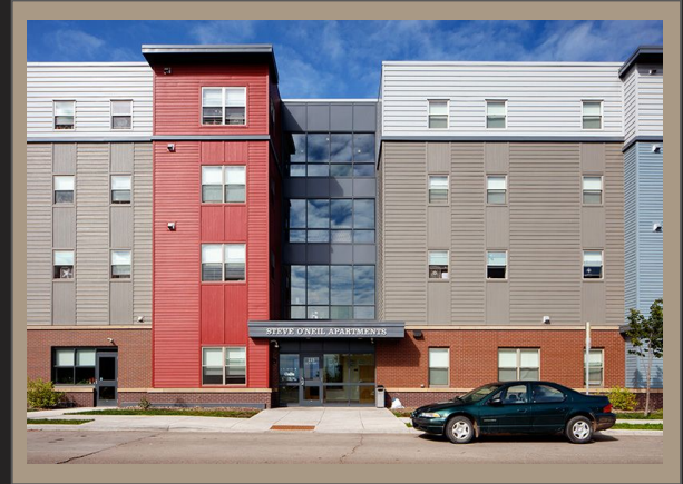
The SONA apartment building
