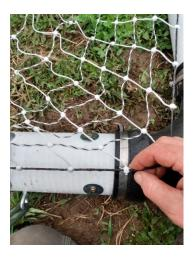
7-Take a fiberglass post and weave it, starting from the bottom of the netting, straight up. Don't clip the top strand to the post cap yet. First, install the black clip, which secures the bottom strand to the spike. You may need pliers or a hammer to make this happen. Be sure that the clip is holding the netting to the spike.
