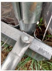
2- Take the 14-foot pipes to the back corners of the HenPen. Place one end of the pipe on the first union on the back and one end on the first union on the side. Attach the bracing to the unions with lag screws. You will be drilling into the wood that you placed inside the union. Repeat this on the other back corner.
