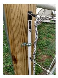
6- Stretch the bottom of the fence along the pipe to the corner until it's taut. Determine where in the netting the next fiberglass post will go. To do this, find the space between the vertical strands in the netting that's as close as possible to the curve of the rubber elbow. Likely, one spike will go through the rubber elbow and one will go through the pipe. Both spikes need to go into the wood at the corner.
