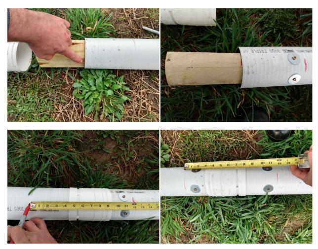
7- Repeat this process until you've connected seven pipes running straight. After seven straight pipes, add a corner as you did before. On the corners, always use non-PVC ends of the pipe to connect to the elbow. You will have to cut the PVC off of a couple ends to make this happen.
