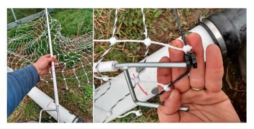
8- Use the fiberglass post to help pull the netting taut again. Press the spikes into the elbow to leave indentations. Drill as you did for the previous post and hammer the spikes in.
