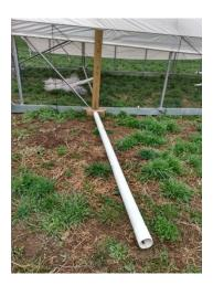
2- You are now at your first corner. Slide a 12" chunk of timber into one end of the rubber elbow until it hits the inside of the corner. Don't force it into the corner. Set the elbow and wood next to the pipe so the end of the pipe lines up with the rim of the elbow, just behind the hose clamp, as pictured. Draw a line on the pipe where the timber ends.
