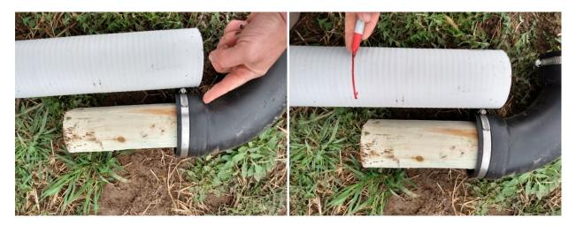
3- With the timber already in the elbow, slide the timber into the pipe. The pipe will slide into the sleeve of the rubber elbow. The red line now indicates where the timber ends inside of the pipe. With fender washers, put two screws through the pipe and into the timber, roughly an inch from the red line. With a 5/16 hex bit, tighten the hose clamp to secure the elbow to the pipe. Put two screws with fender washers through the sleeve of the rubber elbow into the wood.
