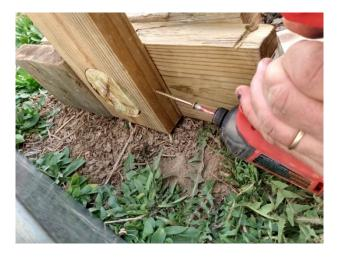
Put a screw through the back of the vertical piece, into the 16" piece. Continue to screw all of the pieces together as pictured. The 5.25" pieces go next to the vertical piece as supports against the baseboard. Be sure to screw them into the 16" piece before placing the whole unit against the base board.
