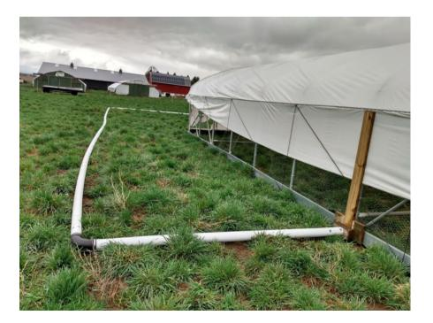
To finish the base of the frame, I set up some simple bracing made out of top rail from chain link fence. At the back of the coop, I bolted the top rail to the base board of the coop and the pipe union, which was ten feet out from the coop.
