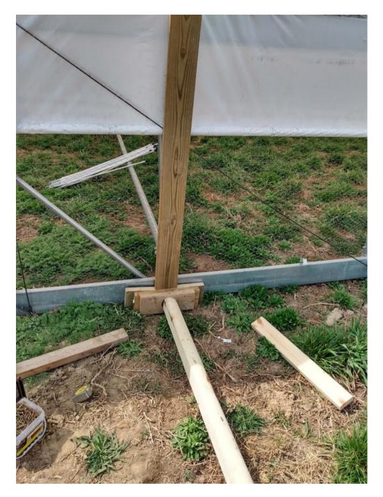
I then added additional layers of 2x6 material at the base, cut a hole large enough to fit a landscape timber, and installed the 8-foot timber, going perpendicular to the coop. The next step was to slide a 4-inch UV-resistant HDPE pipe over the landscape timber. After I secured the pipe with screws, I added an 18-inch chunk of timber to the open end of the pipe, secured it, and added a rubber 90-degree elbow with the open end pointing toward the rear of the coop.
