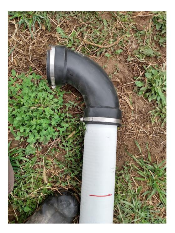
At that point, I continued to lay out seven pipes straight back and connected each of them with a 12-inch chunk of landscape timber. When all seven were connected, I added another corner. The rear of the fence base consisted of four pipes, then I repeated the first side to complete the system all the way over to the other side of the coop where it would attach to the other mount.
