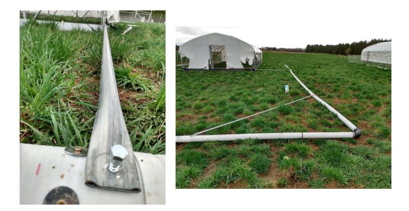
Then I made a 14-foot piece of top rail and bolted it to each union ten feet from the back corners. This helped maintain the shape of the frame when the coop moved. Now it was time to attach the poultry netting. First, I took all the posts out of the fence, and cut the tips of the spikes down to 3.5 inches.
