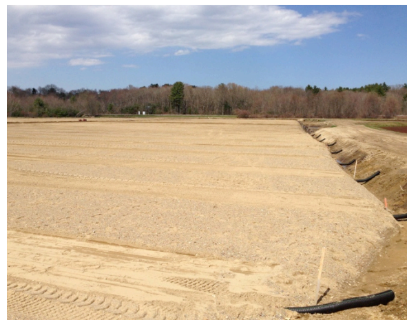
Finished grade showing tiles extending out of keyholes.
