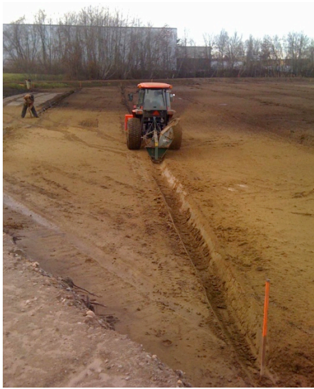
Trenching in a keyhole for tile in a renovation.
