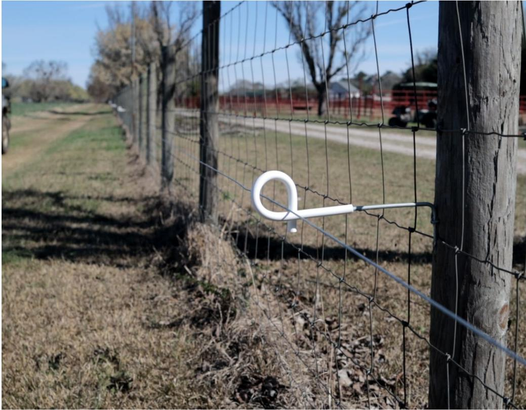
Figure 2: Perimeter fence of Woven Wire with Pigtail Extending 5” out from Post, approximately 24” off the ground.
