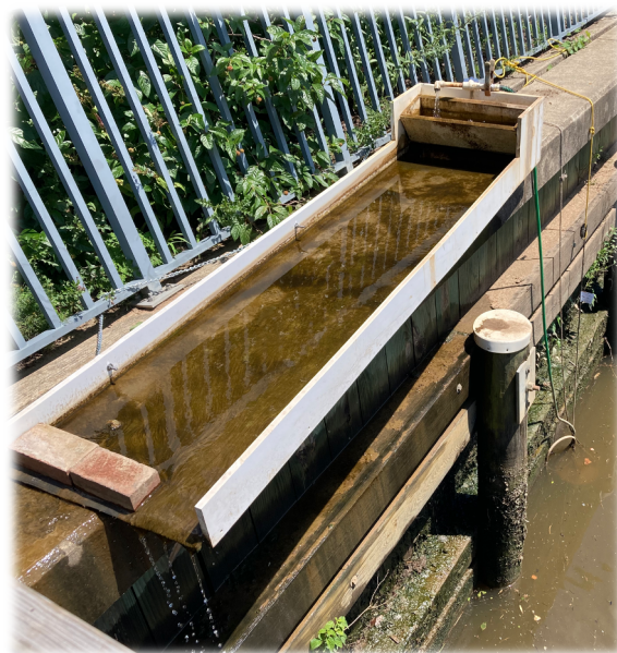
Figure 1: An example of an algal turf scrubber, or ATS, installed on the Anacostia River at a park in Bladensburg, Maryland.
