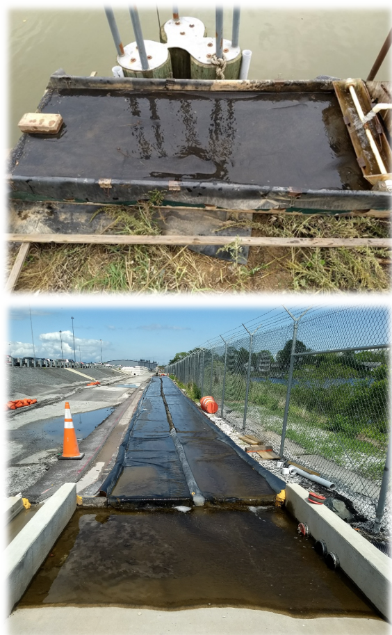
Figure 2: The size of an algal turf scrubber can be customized according to the space available at a site, from small dockside units (top) to large commercial systems (bottom). Nutrient uptake and the volume of algae grown increase with surface area.
