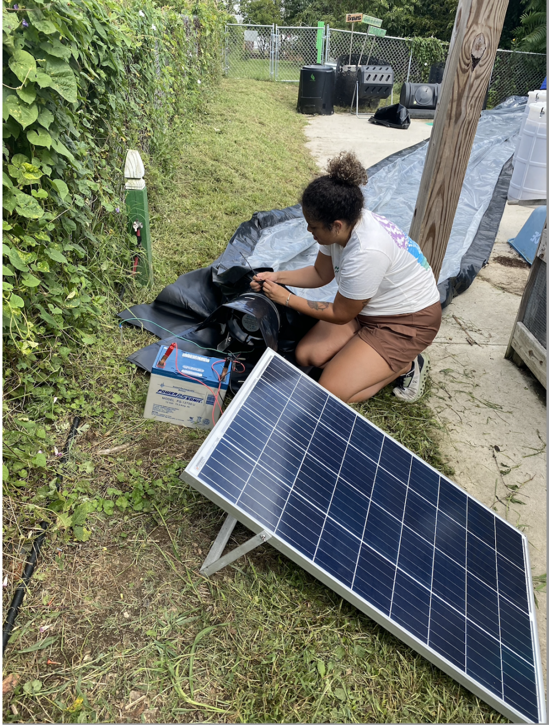
Figure 9. Wiring the motor to the solar power battery.
