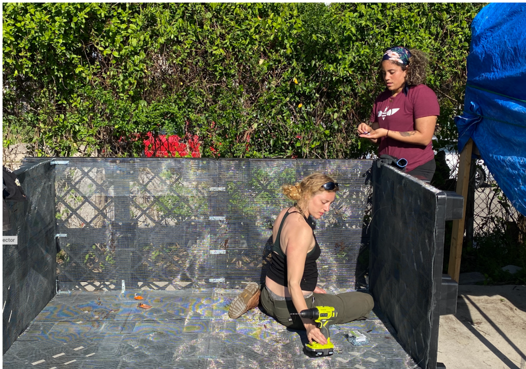
Figure 4. Installing hardware cloth in the interior lining of the containers.
