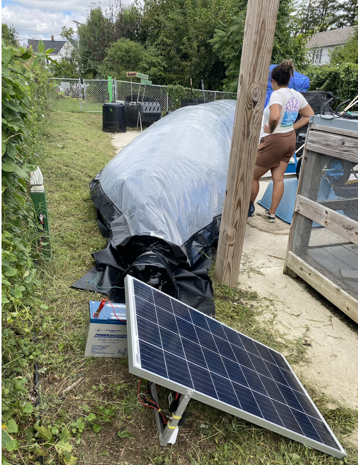
Figure 8. Connecting a solar panel and battery to build off-grid resilience into the production process.
