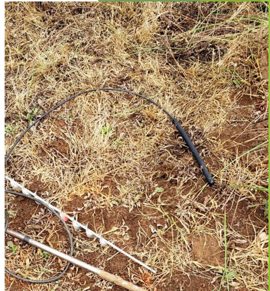
The DRI deep drip units can be seen here installed and connected to the incoming row supply line.
