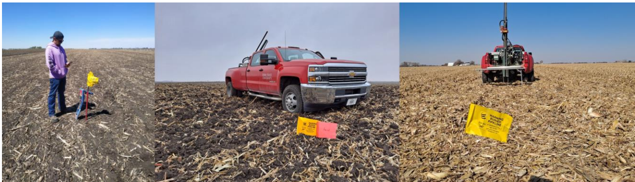
Fig. 2. Demarcation of pipeline path before sampling
