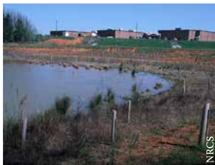
A constructed wetland treats wastewater from a processing plant.
