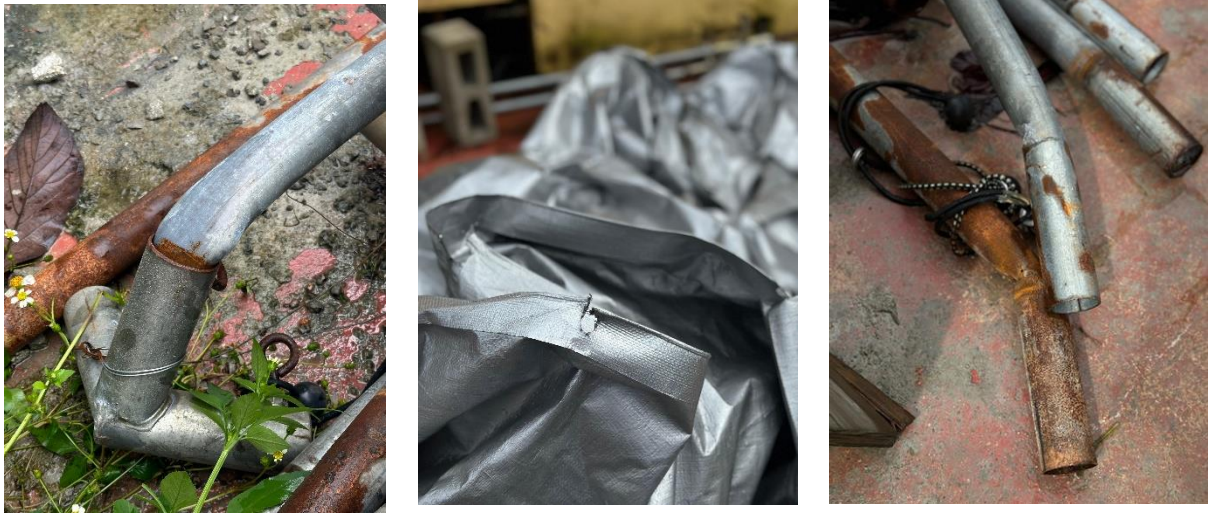
Photos of damaged canopy stands and tarps from the heavy rains in Guam. Sept-Nov 2024
