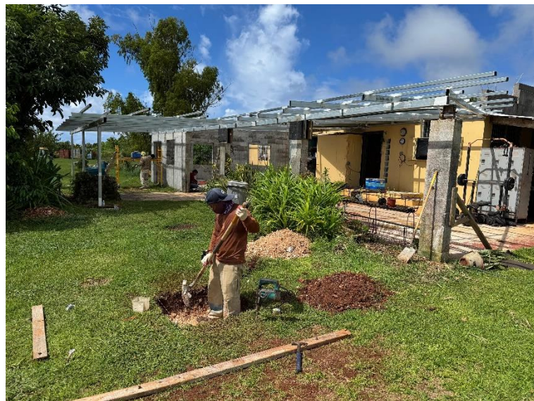
Ongoing work at the research jobsite to improve and build resilience.
