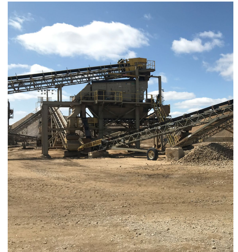
Affgregate Industries Empire Plant is a high-capacity sand and gravel operation that manufactures aggregate products for ready mixed concrete, precast concrete and asphalt applications (Photo courtesy Mike Krcmarik, NRCS)
