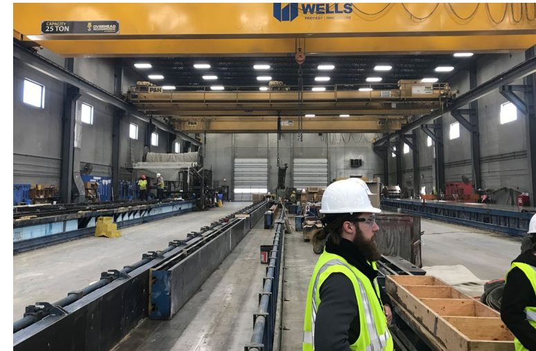
The Wells Rosemount precast concrete production facility opened in 2016 and currently produces structural members of prestressed concrete including double tees, beams, columns, and stadia. (Photo courtesy Mike Krcmarik, NRCS)
