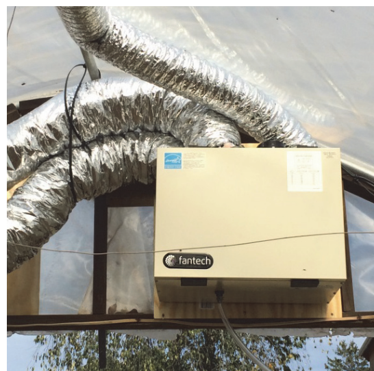
The 106 CFM Fantech heat recovery ventilator installed in the gable of the lower high tunnel (LHT) at New Morning Farm. Photo: Chris Lent, NCAT
